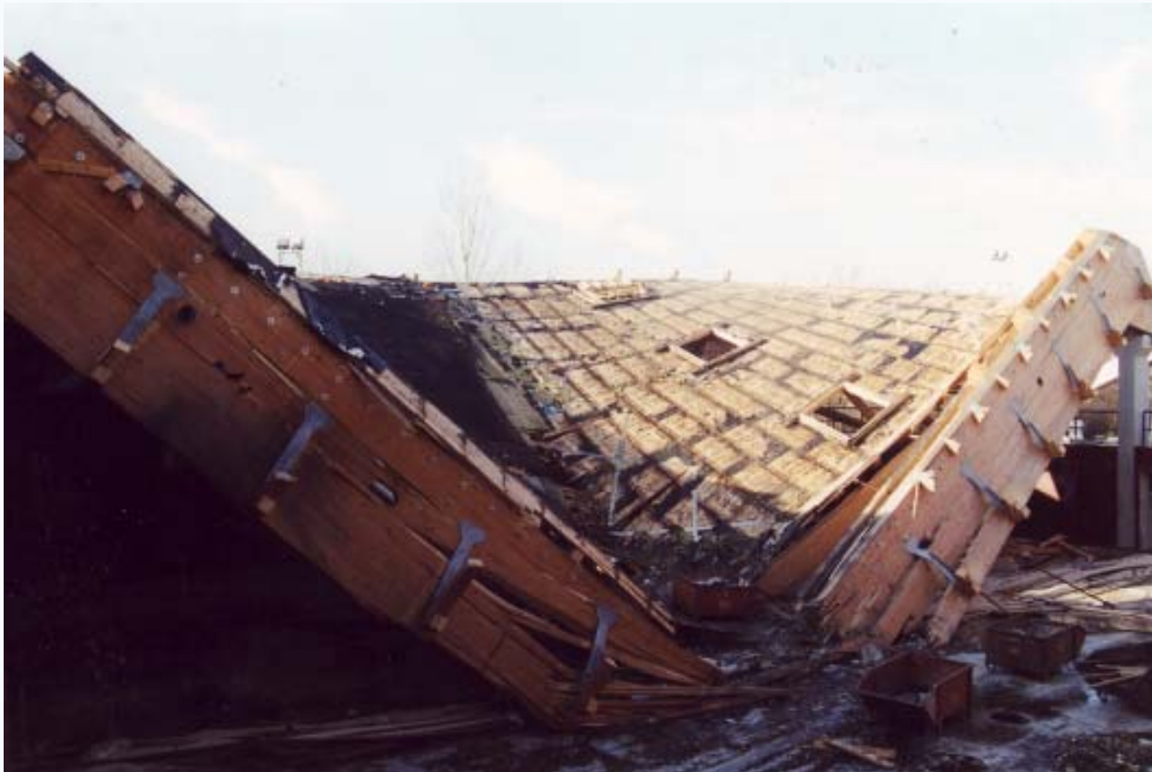
Gymnasium, sports hall, 2000
