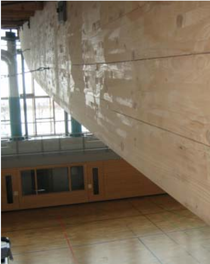
Cracks – changing of moisture
